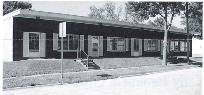
Work will begin later this summer on the new Vera French Outreach Center. Remodeling expenses will be funded by donor support: Please contact us to see how you can be a part of this!
